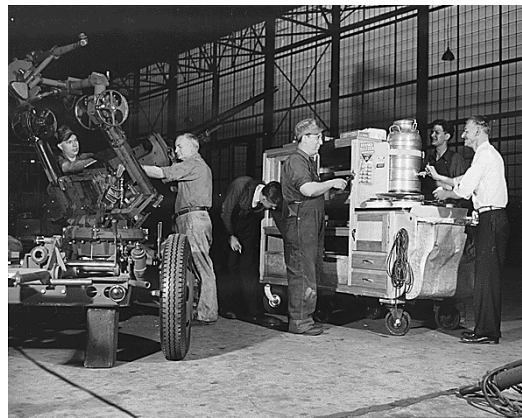
Assembly of 37mm Anti-Aircraft Guns Picture Source: FDR Library Archive
